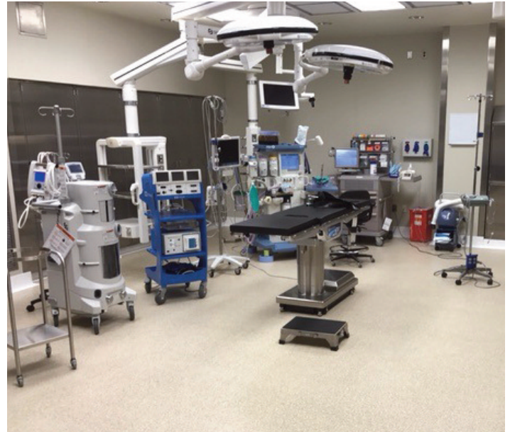
A poured-in-place urethane mortar system provides this orthopedic surgical suite with weldless, long-lasting, stain-resistant floors.
